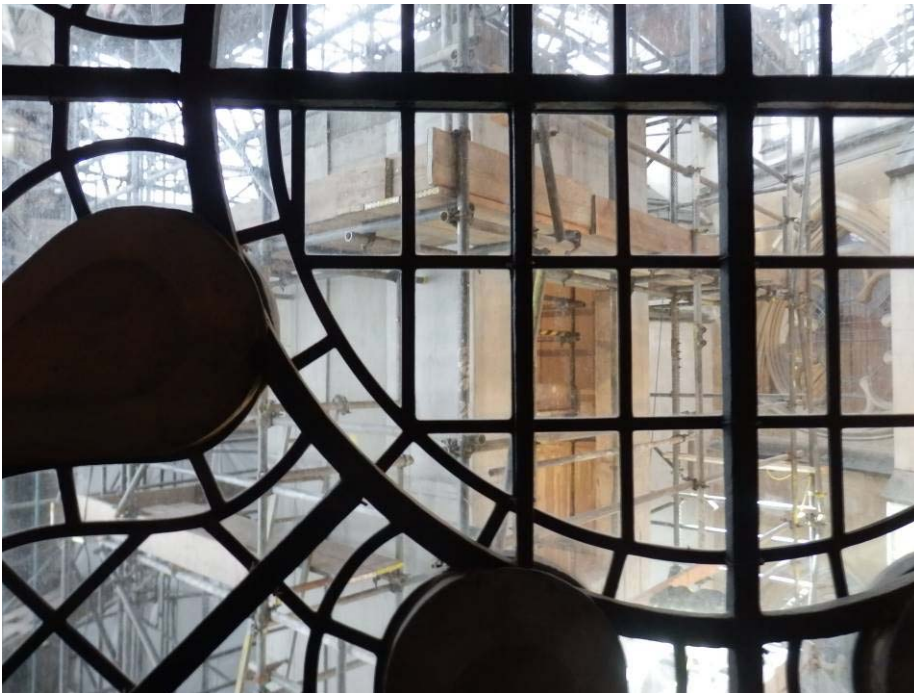
The new tower under construction seen from inside the Triforium gallery
