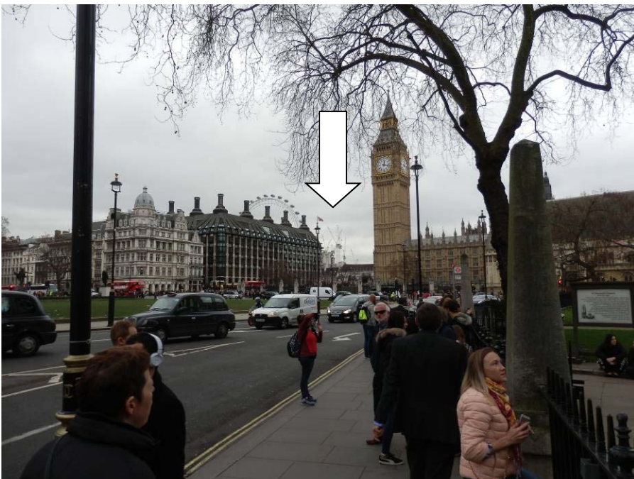
From a larger distance: Shell Centre construction cranes near Elizabeth Tower. The new building is going to narrow the "gap" and diminishes the vertical accent of Elizabeth Tower.
